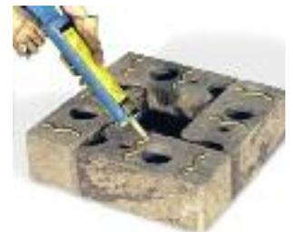
Secure the blocks together with masonry adhesive to add strength to the post/pillar
