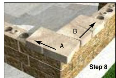
Secure the Wall Caps in place with a bead of masonry adhesive along both sides of the raised rings and along the sides of each Wall Cap.
