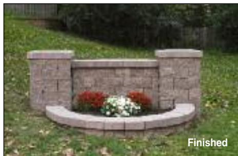
Once all the caps are installed, secure them in place with a bead of masonry adhesive on both sides of the raised rings. Then add any additional soil you may need to fill the planter area. If you would like to add lighting to your project, see **How-to Sheet #170 for information on how to construct a light post.**
