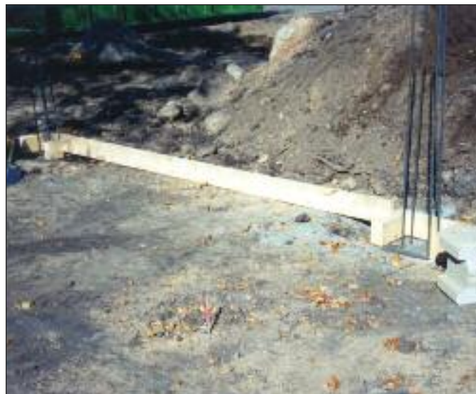
Figure 1: AB Fence Pile Layout Jig
