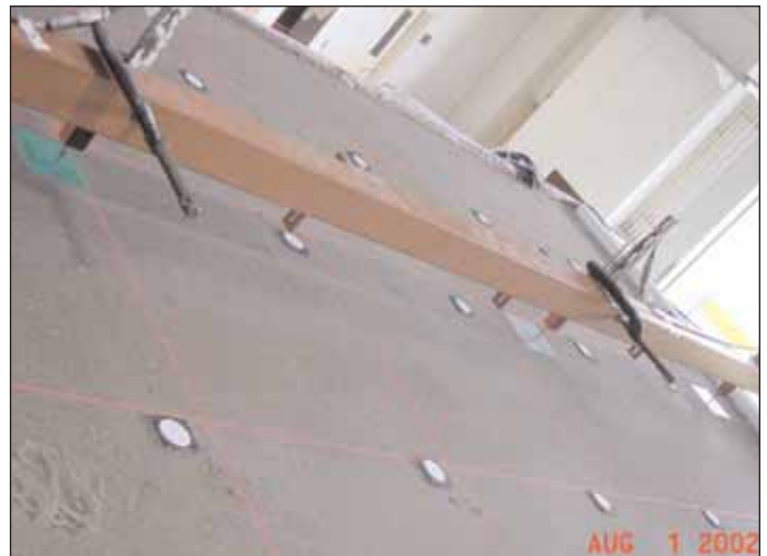
LVDT and Markers on the Backfill Surface
