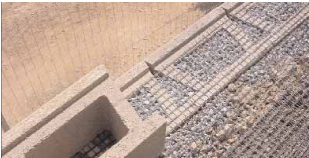
Allan Block reinforced with Huesker geogrid.
