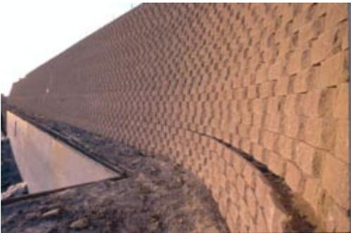
The design of the retaining walls required involvement from all engineering parties contracted for the project. The site civil engineer determined the height requirements for each wall. The south group of walls were the cut walls with maximum heights of 50 ft (15.2 m) and the north walls were the fill walls with maximum heights of 25 ft (7.6 m). The retaining walls at the Jewish Academy were subject to active soil pressure from the native sandy soils.
