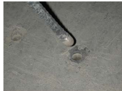
Figure 5: Footing Dowel Insert
