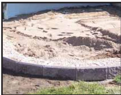
Make minor adjustments by using a dead blow hammer or by placing up to 0.5 in. (13 mm) of course sand under the blocks. Keep in mind irregularities in the base course become larger as the wall stacks up, causing your patio to be uneven. Paying extra attention to your base will ensure your wall is level.
