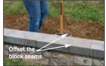
AB Courtyard can be built taller than two courses, but only a maximum height of two block courses can be used to retain soil. For added stability options, see How-To Sheet #150 or to retain soil taller than shown here, see our Retaining Walls Installation guide for walls up to 6 ft. (1.8 m) tall using our retaining wall products at [allanblock.com](http://allanblock.com).
