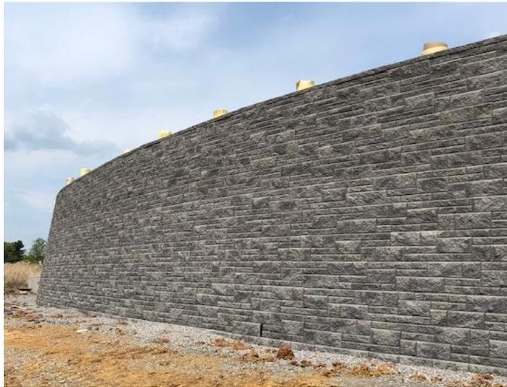
design process easy. These walls are partial cut-and-fill walls due to the regrading of the site. Mike used Stratagrid 200 at a 2-course block spacing which is the National Concrete Masonry Association’s (NCMA) best practices suggestion that builds a very solid reinforced soil mass.
