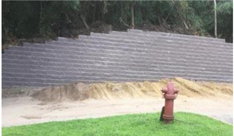
wall using geogrid. By using no-fines concrete the infill area was a fraction (up to a 50% reduction) of what would be needed for a typical geogrid application. This leads to less excavation which accommodates the site constraints above the wall, such as existing trees.
