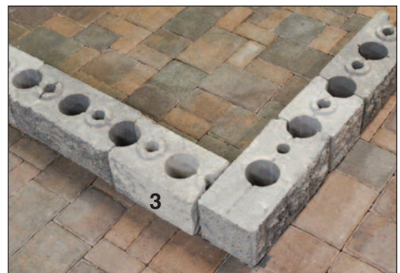
Build Wall Panels
