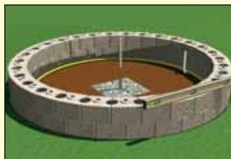
Excavate the area outside the liner 3 in. deep (75 mm) and 8 in. (200 mm) wide. Fill in the trench with wall rock, level and compact.
