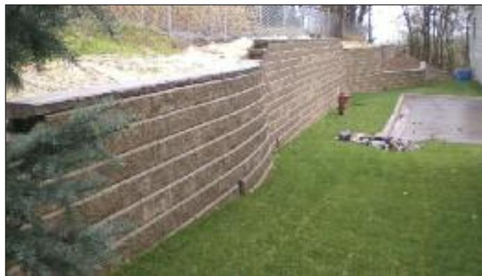
No-Fines concrete has been utilized in the construction industry for decades and the segmental retaining wall industry for more than 15 years. Like most concrete mixes, No-Fines concrete includes portland cement and coarse aggregate. However, sand (fine aggregate) is omitted from the No-Fines mix to allow voids
